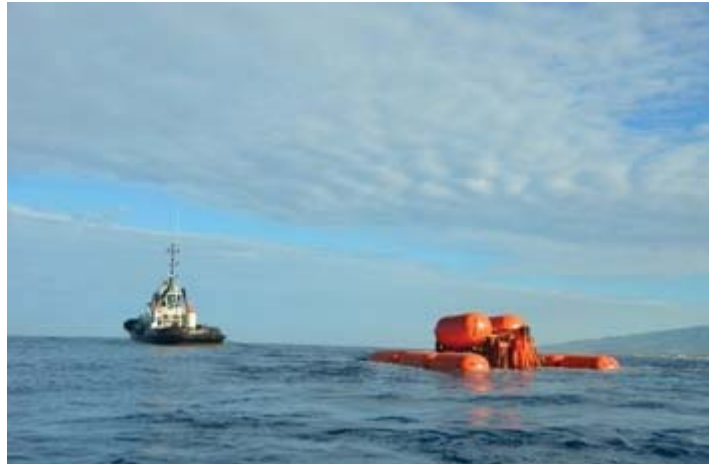
Figure 5. Tow-out of the subsea energy management system at Reunion Island
